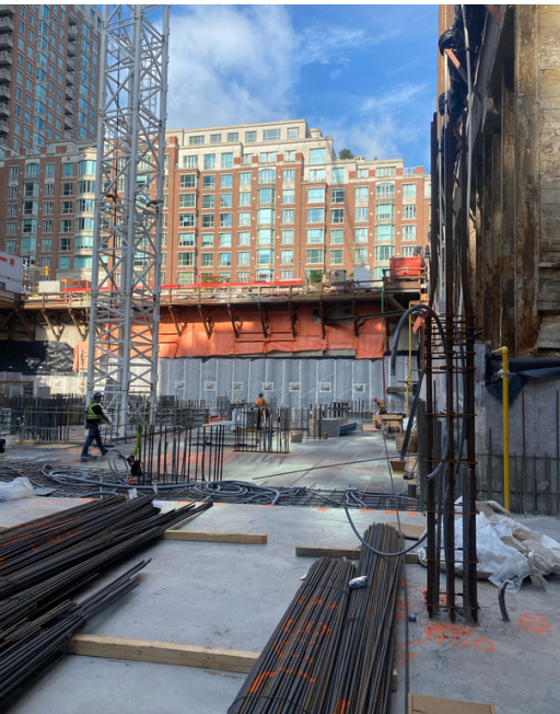
(Figure 2): Progress of level P2 looking West.
