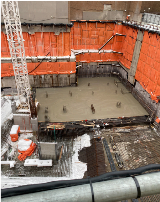
(Figure 2): View of concrete poured at the NE corner of site.
