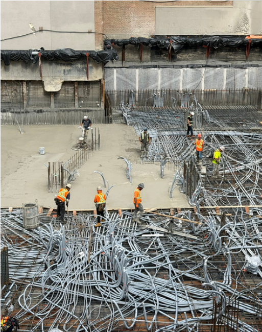
(Figure 2): Progress of the concourse level slab pour. View of North elevation.
